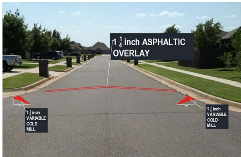
EDGE MILLING AND THIN OVERLAY (1 1/4')
