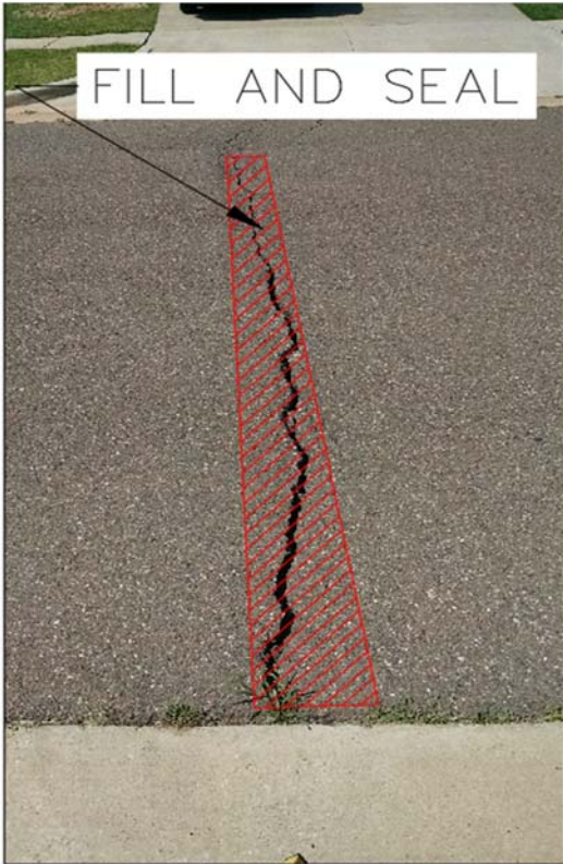
MAJOR CRACK REPAIR
